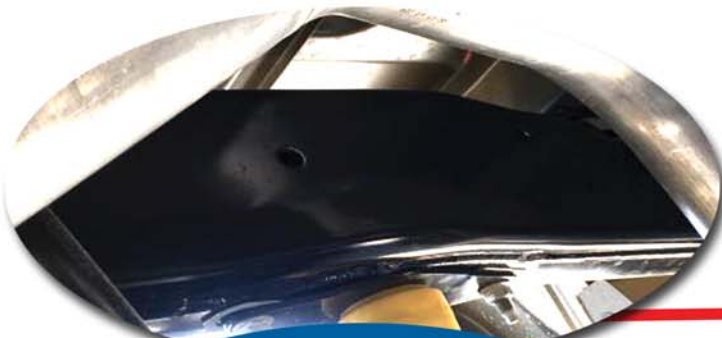
Picture shows 'No' inner side plates welded on frame. New Style
